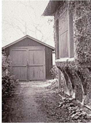
BIRTH OF A NOTION: The one-car shed at 367 Addison Avenue in Palo Alto was the company's workshop and launching pad in 1938.
