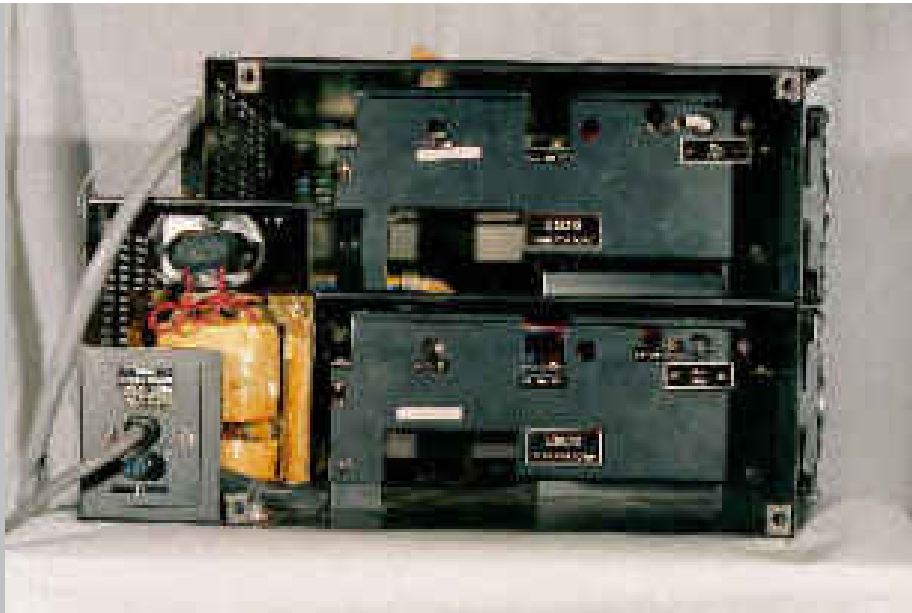
PDP-8/A 620 The Rear of the Cabinet.
